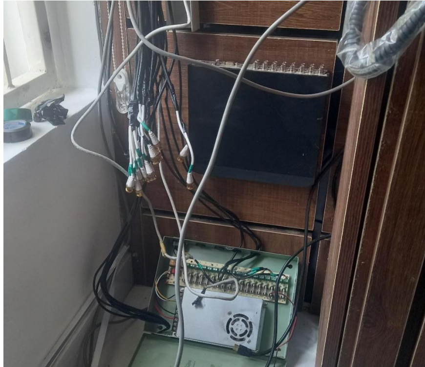
FIG 18: CONNECTING THE CABLES TO DIGITAL VIDEO RECORDER
